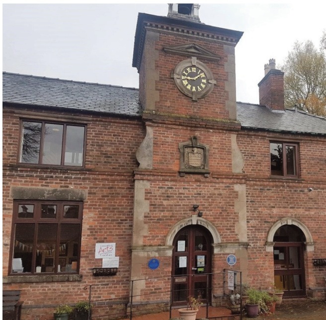
The renovated Clock Tower Building
