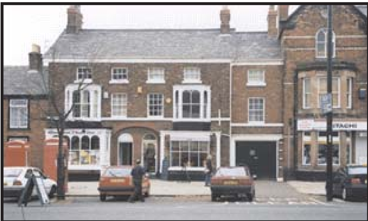
Millmark on the left c.2000, formerly the Telephone Exchange
