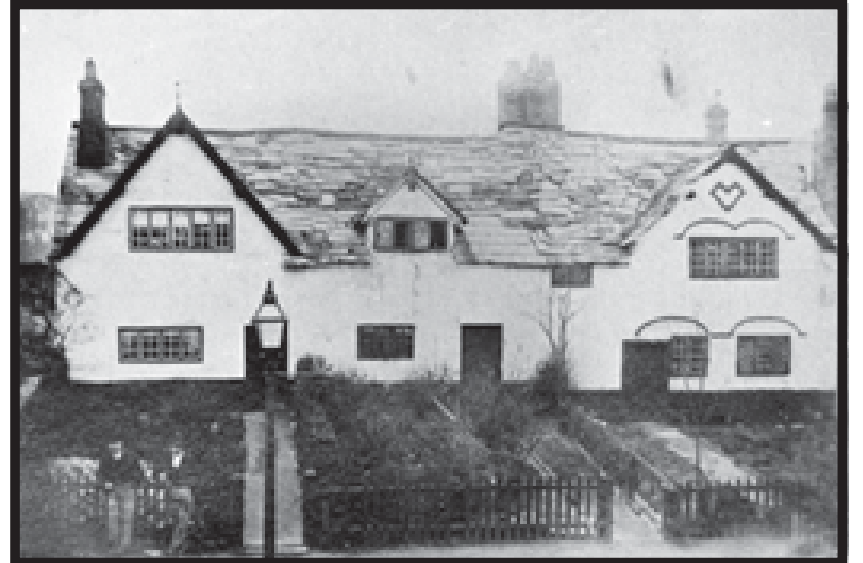
The Church St cottages demolished in 1878
