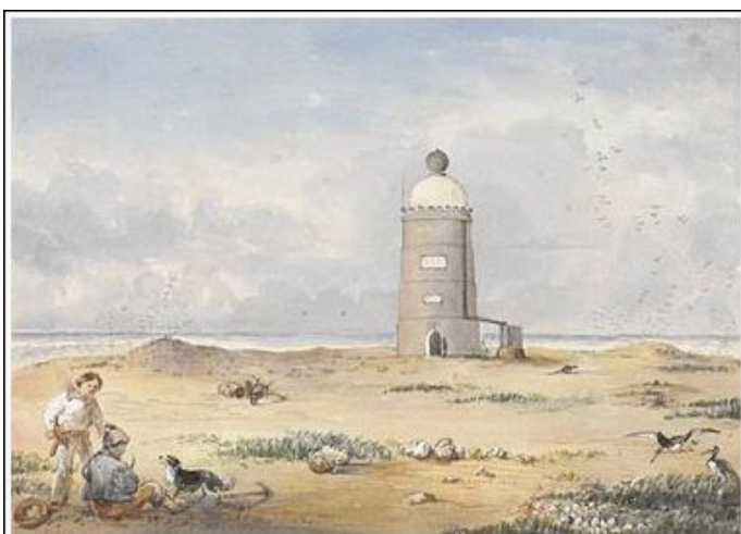
Beacon built at Raines Islet by Edwin Augustus
