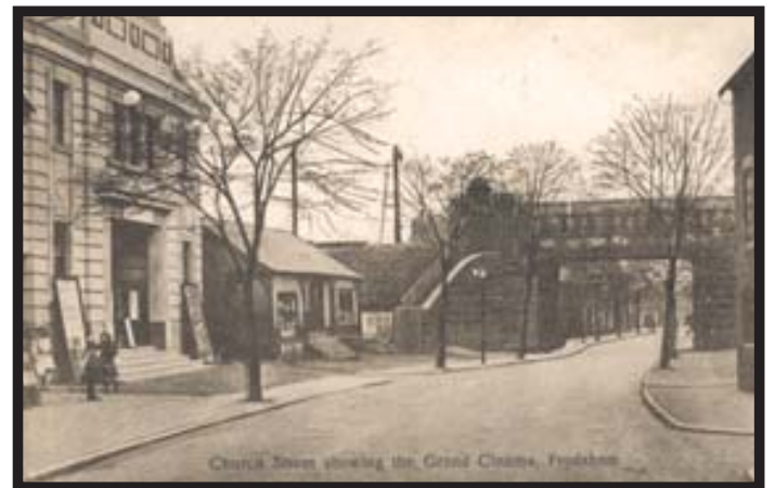
Reused cricket pavilion c.1930s
