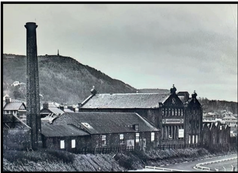
Kydd's Jam Factory prior to demolition
