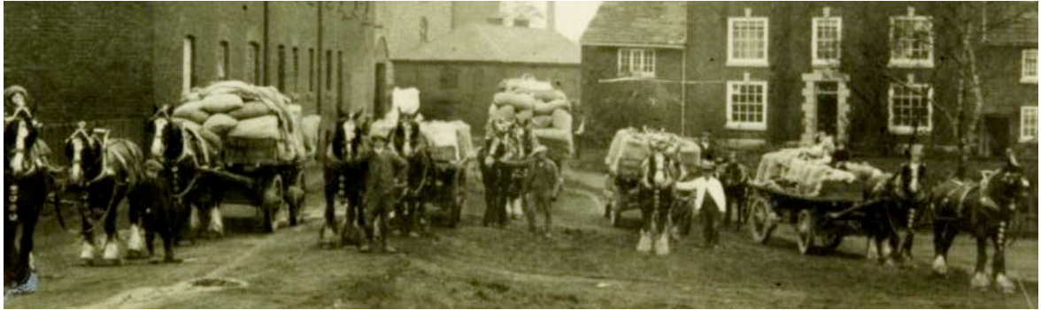
Thomas Rigby's Mill. Grain arrived by barge then via an elevator to the top floor raised at 60 tons/hour
