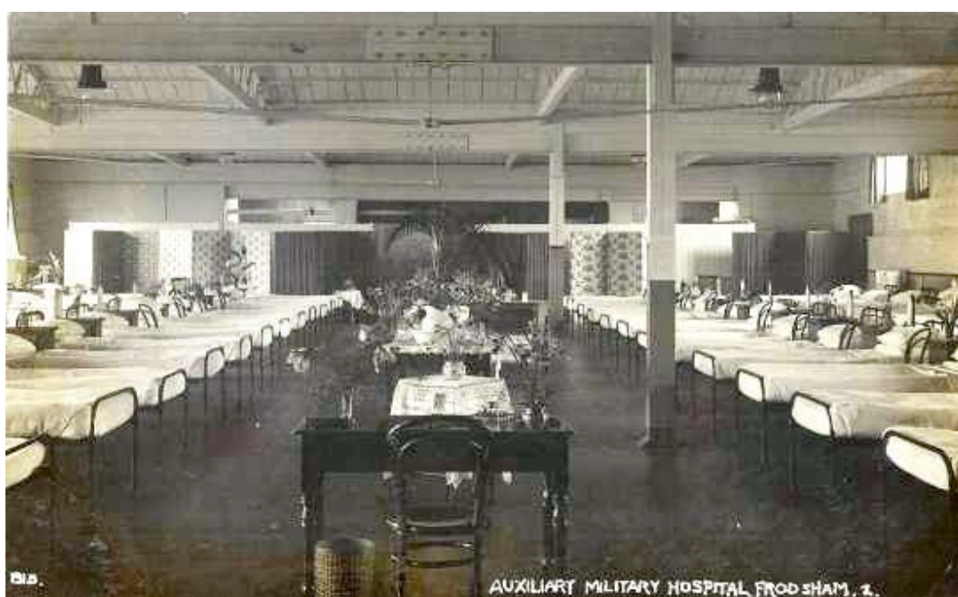
The interior of the 30-bed Auxiliary Military Hospital in 1915
