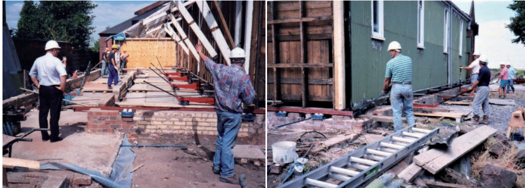
The 'Iron Church' being moved 3 metres sideways in 1995
