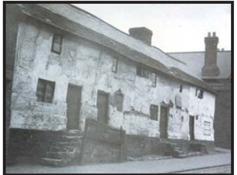
Old cottages prior to demolition
