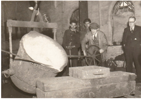
E. Timmins & Sons, Bridgewater Foundry, Runcorn Image courtesy of R&DHS, Arthur Timmins Archive- copyright.
