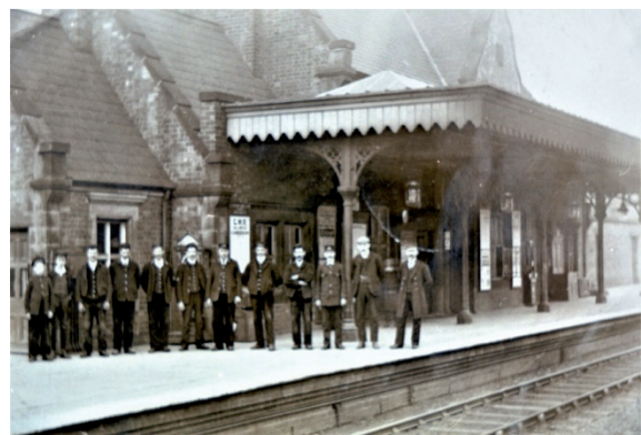
FDN0936 - Canopy built over widened platform c.1900
