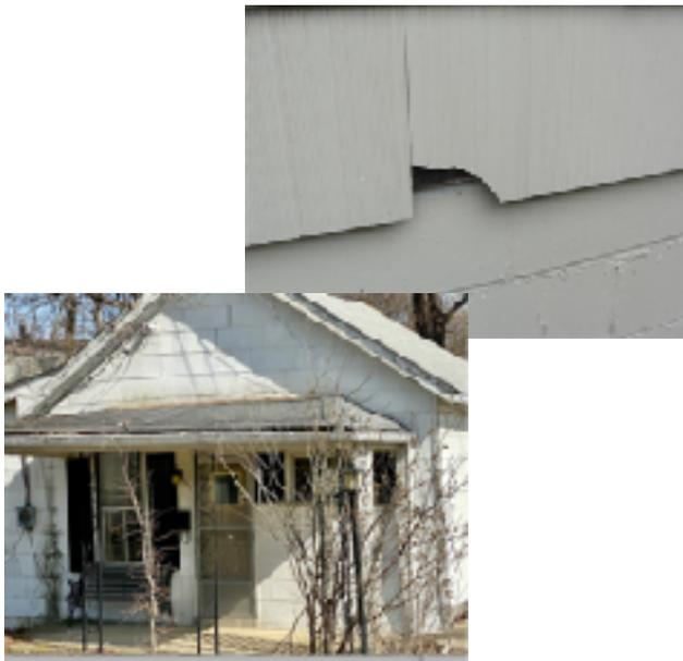
What about asbestos siding, which many older homes were sided with up until about 50 years ago (when it was banned in the U.S. for health reasons)? Asbestos siding can be quite fire and heat resistant. The problem is in the gaps. Older siding such as this often develops cracks and openings as shingles shift and move. Such gaps need to be carefully filled to prevent embers entering and igniting the building. (No gaps larger than 1/8 inch should remain)
