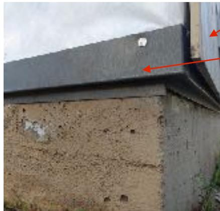
One homeowner's method of protecting bottom of old wood combustible siding with metal flashing.. Consult a contractor for your situation.
