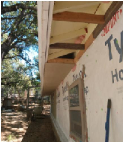
New siding can often go right over old siding, if the wall is sound. A vapor barrier is generally used between the two layers. Pay attention to the bottom of the wall however - metal flashing needs to go over the old, combustible siding where it is still exposed at the bottom. (NIST 2205 Table A Appendix A recommendation)
