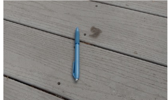
Small burn mark on Azek deck board, with pen for scale
