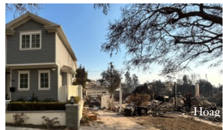
Surviving home right next to destroyed home, Palisades
