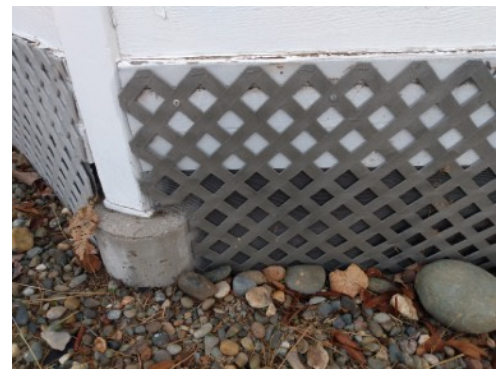
Gazebo: Fine mesh screening behind lattice, plants removed.
