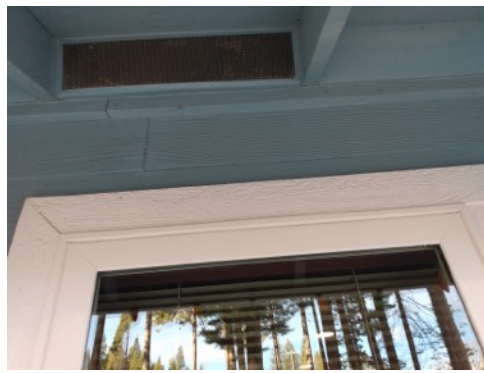
Eaves: No gaps, and Vulcan vents- both fire and ember resistant. New tempered windows
