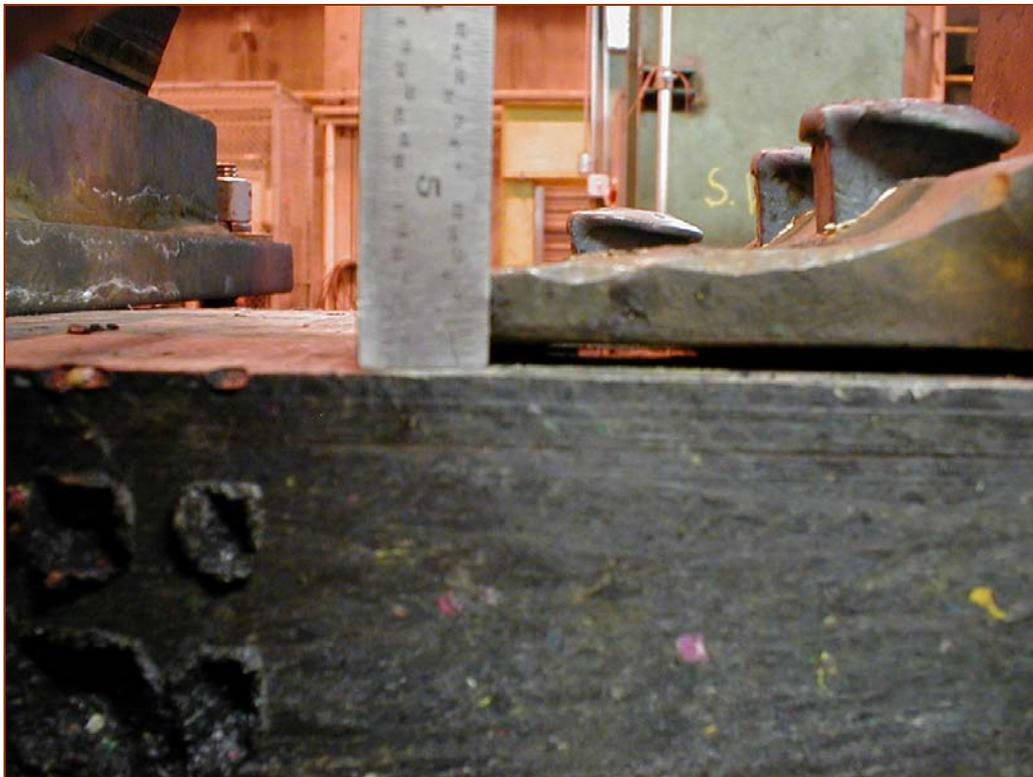
**Figure A-5. Close-up Gap between Tie Plate and Tie**
