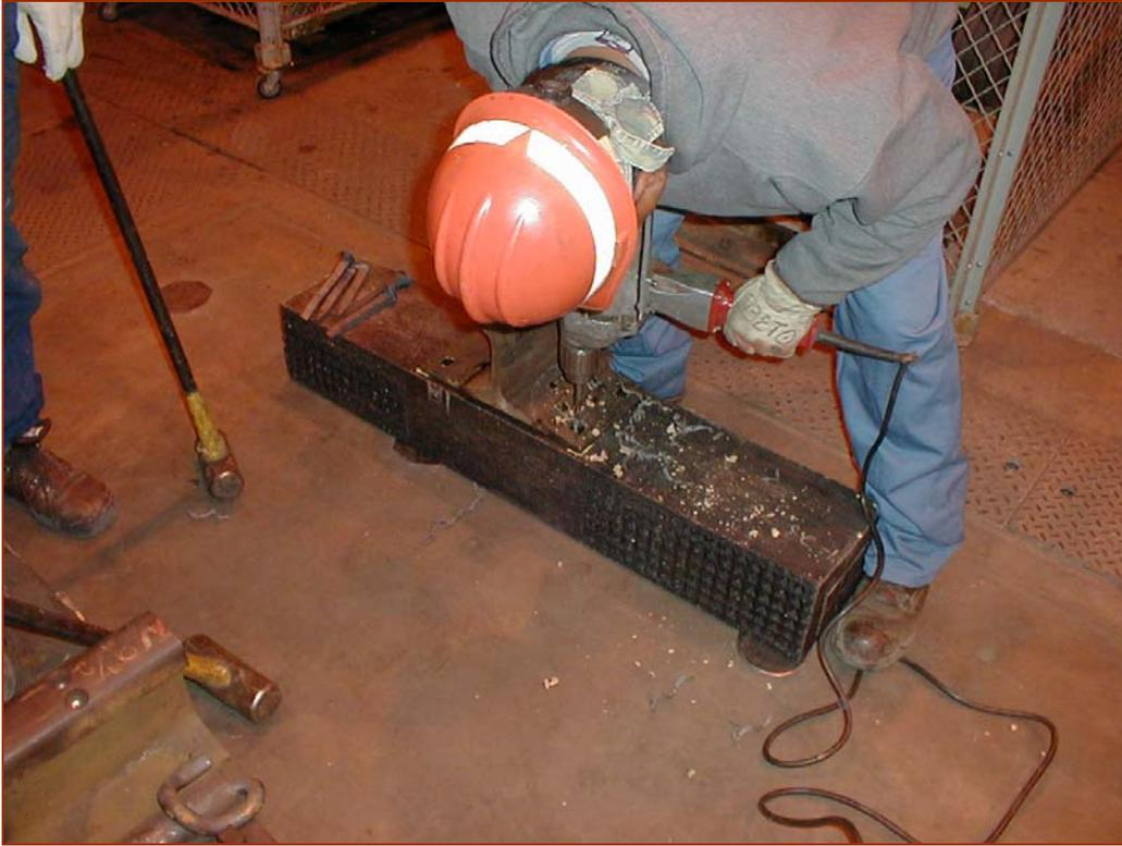
**Figure A-2. Predrilling Spike Holes**
