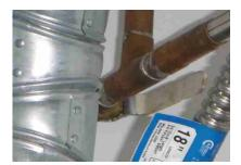
Gas Shut-Off Valve & Connector Informational Conditions The gas control valve and its connector at the water heater are functional.
