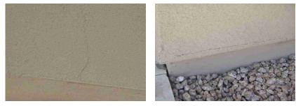
I observed areas where the stucco lath is exposed. Repairs should be made so that the lath does not rust. E.G. Underside of the rear patio. Underside of the front entry.
