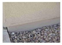
• I observed areas where the stucco lath is exposed. Repairs should be made so that the lath does not rust. E.G. Underside of the rear patio. Underside of the front entry.
