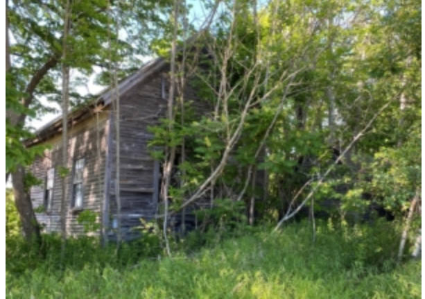
Trees and brush surround the 1867 Pigeon Hill Schoolhouse on Route 26, the last standing one-room schoolhouse in Oxford. The Oxford Historical Society proposes to move it to the Kay House Museum property on Pleasant Street, restore it and use it as a living history museum. Nicole Carter/Advertiser Democrat
