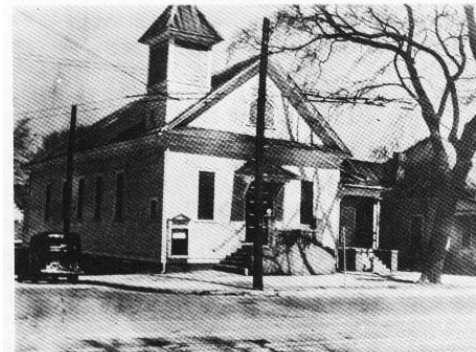
1 st West End Ave. Bldg.
