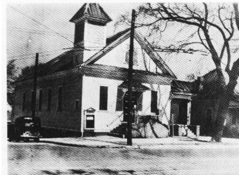
1 st West End Ave. Bldg.
