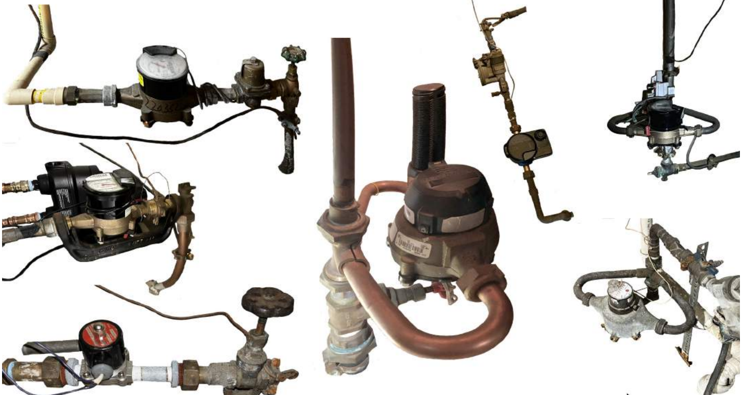
Figure 29. Various Basement Meters and Service Configurations.
