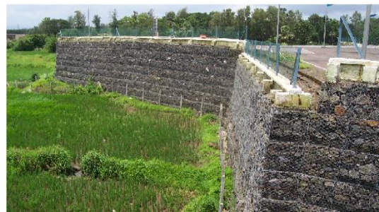
FIG 6- Gabion retaining wall
