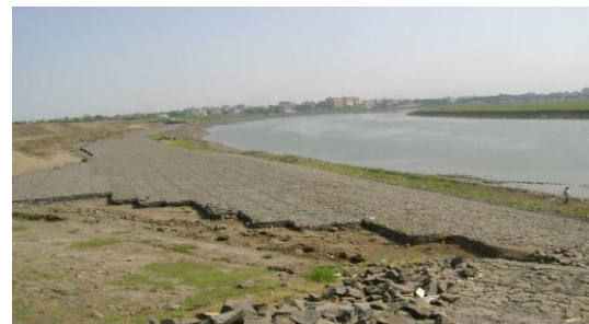
FIG 7- River bank protection
