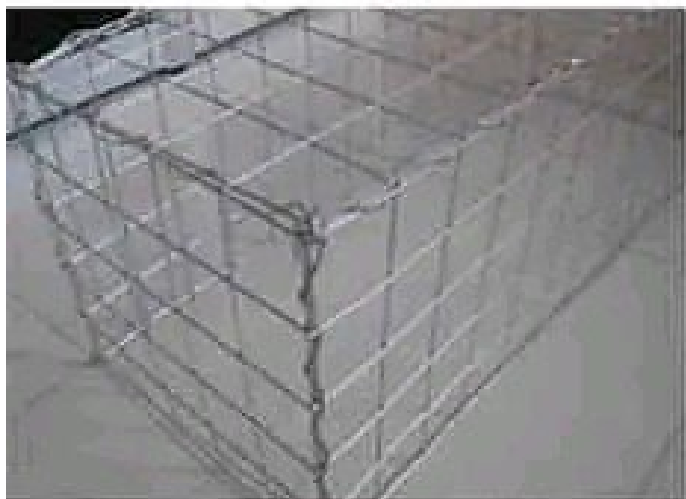
Lacing wire connection
