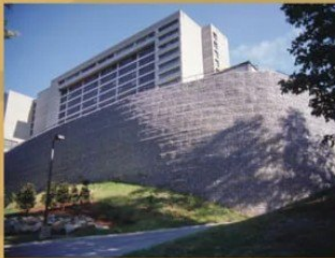
Mechanically Stabilized Earth (MSE) Gabion Wall [Reinforced Soil Wall]
