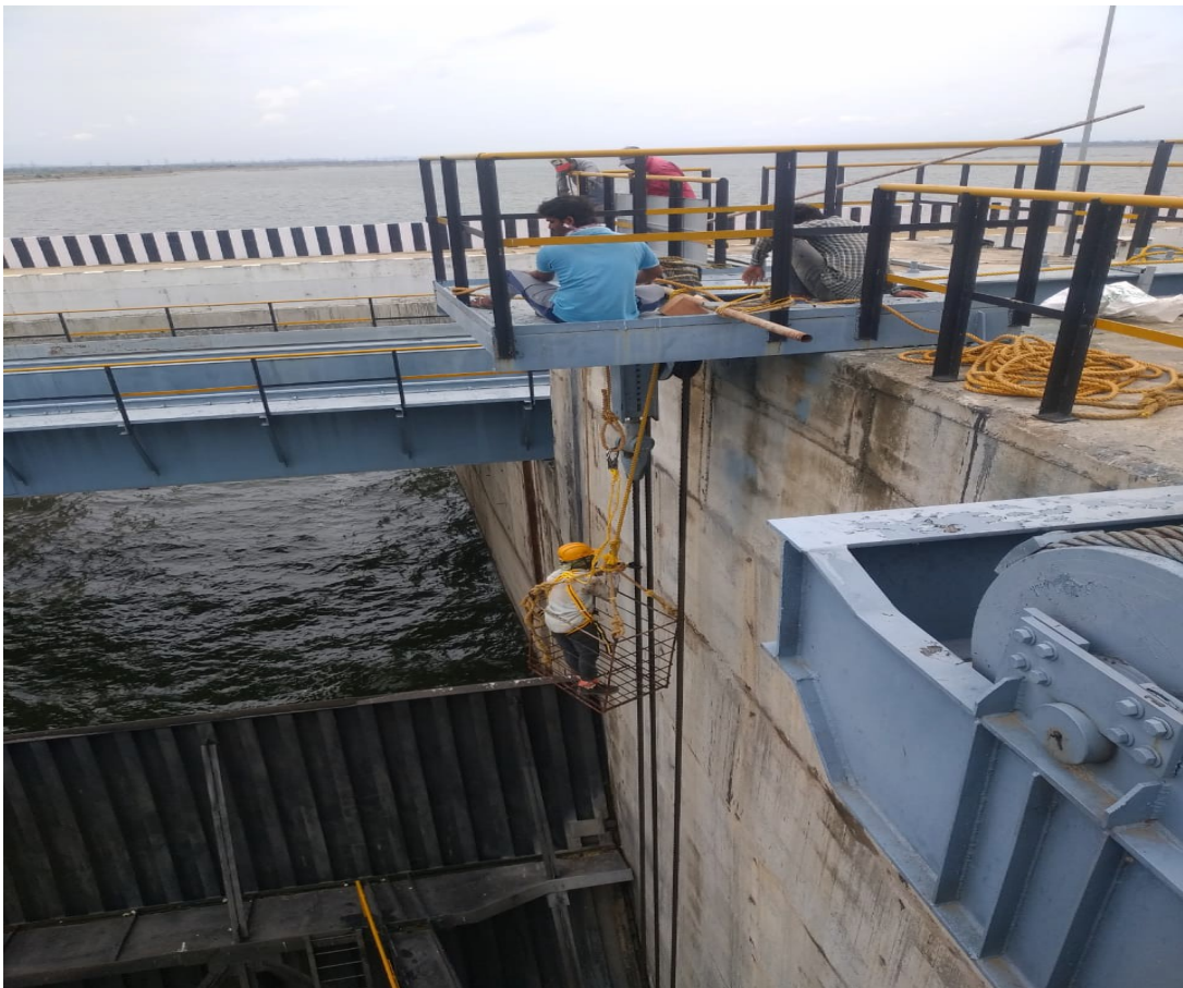
Application of cardium compound to wire rope with brush
