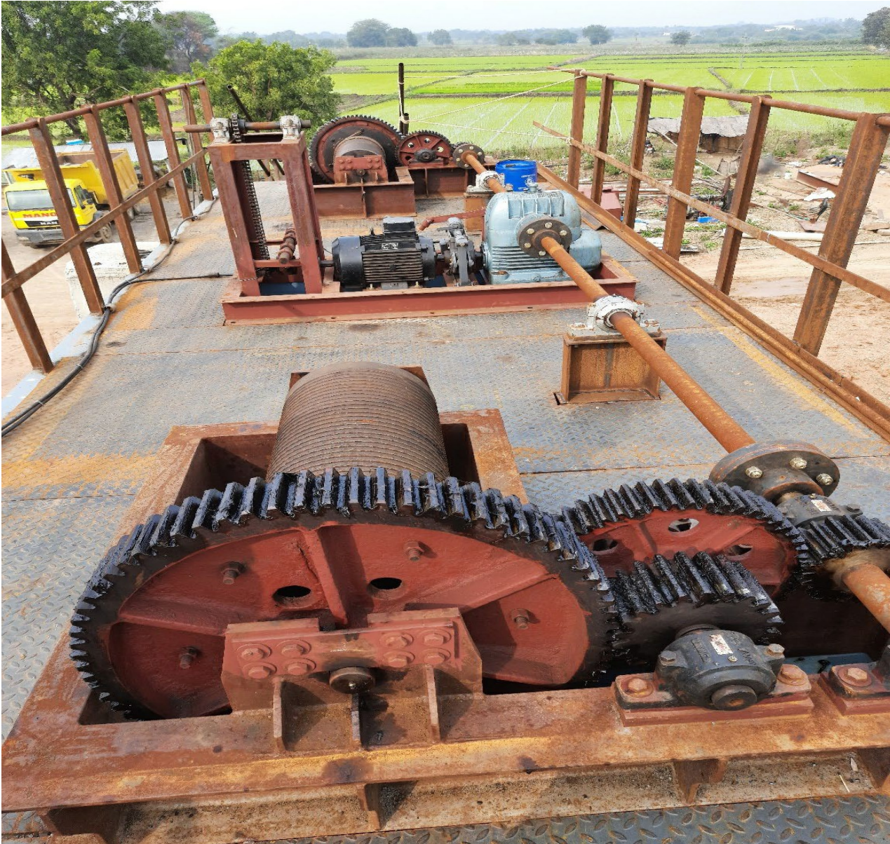
Upstream Rope drum Hoist – Gear Train Assembly
