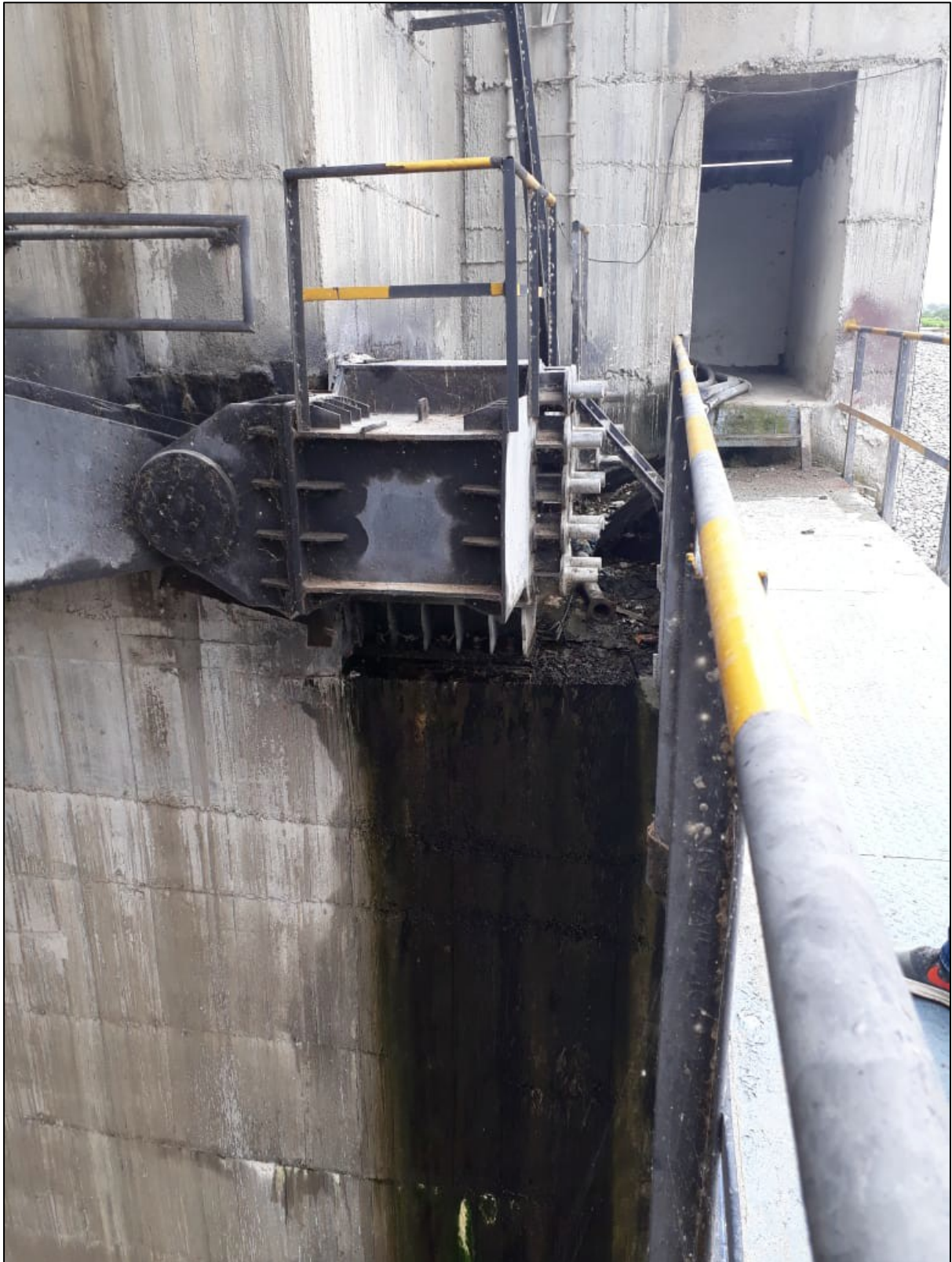
Water Stagnation at vertical chair of Radial Gate
