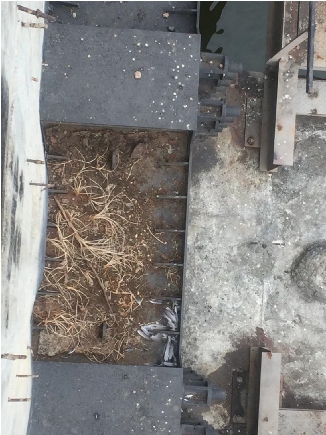
Debris removed on trunnion girder / yoke girder
