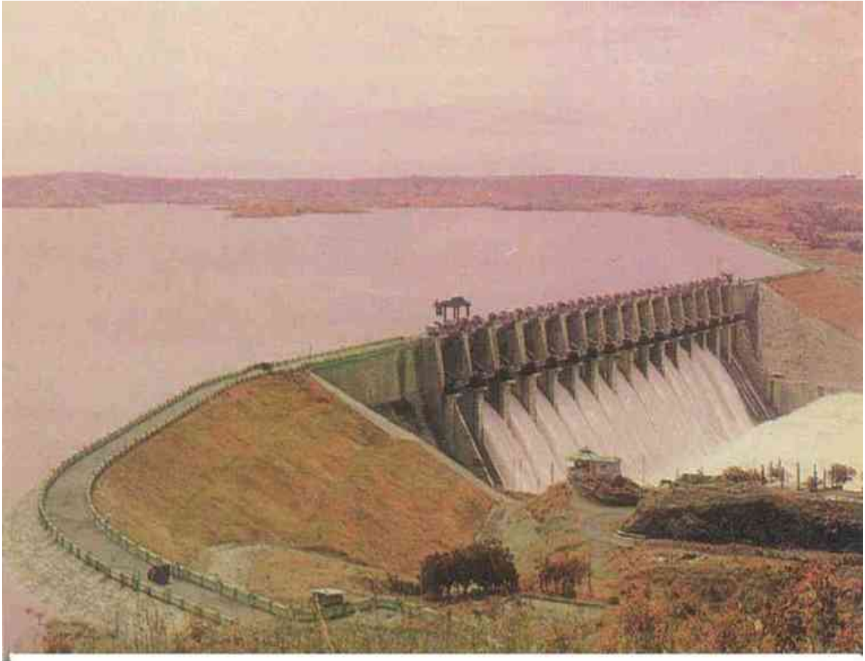
FIGURE 45. Mahi Bajaj Sagar Dam across river Mahi in Rajasthan showing ski-jump bucket energy dissipators in action
