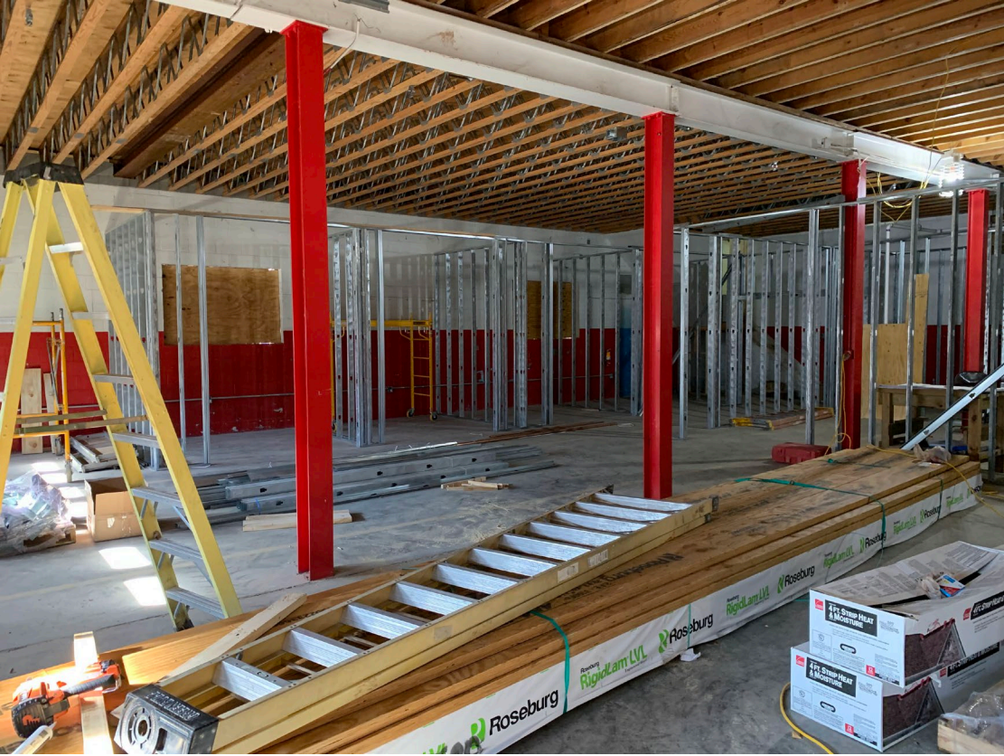
Framing for Offices
