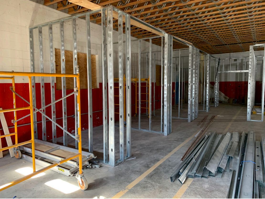
Framing for Offices
