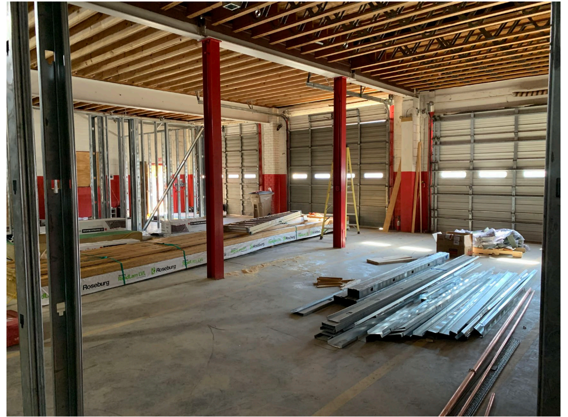
Framing for Conference Rooms
