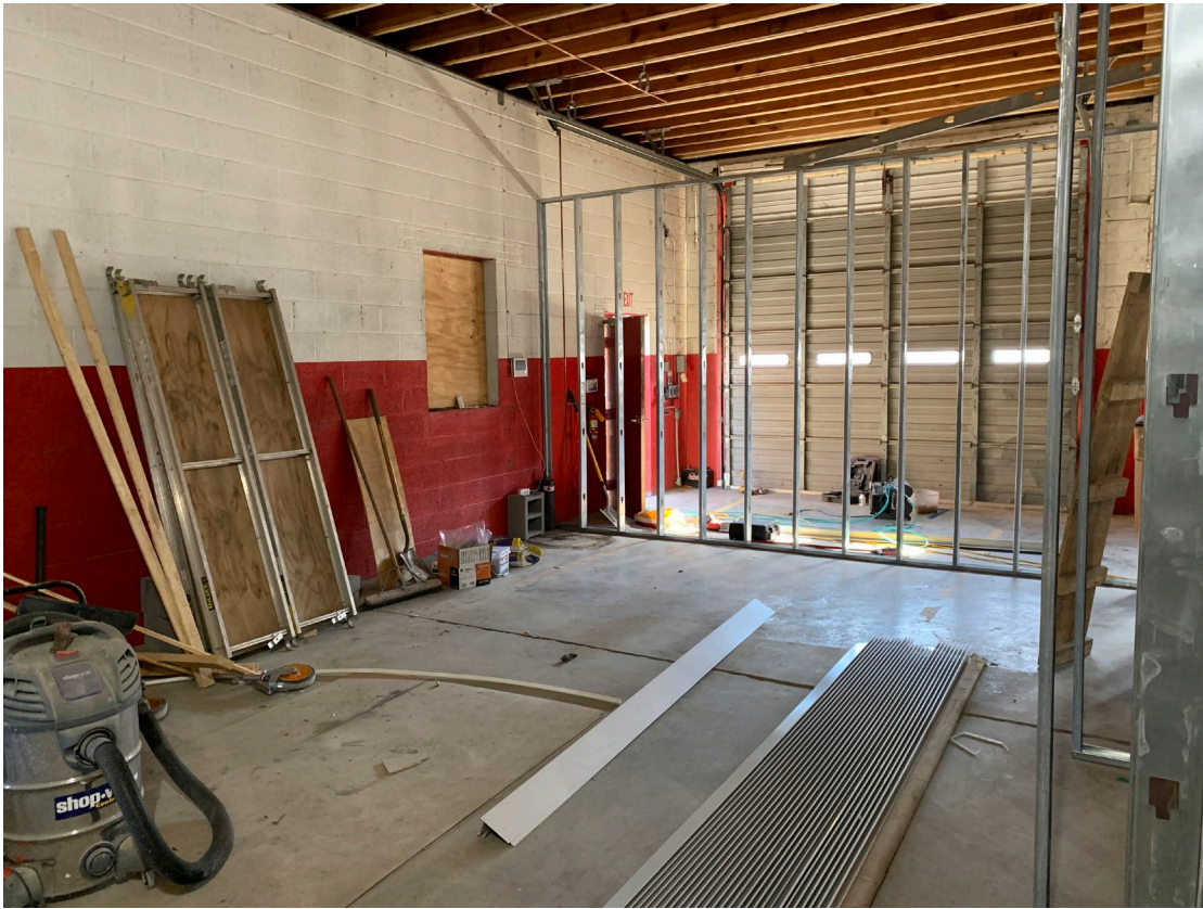
Framing for Conference Rooms
