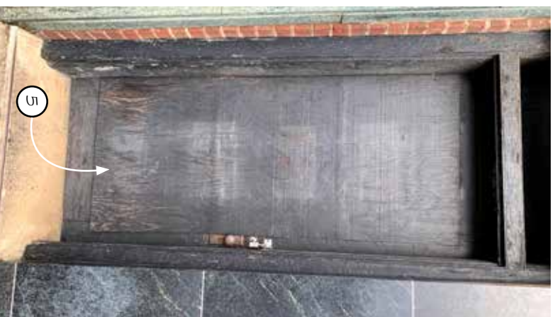
EXISTING SIDE ENTRY
