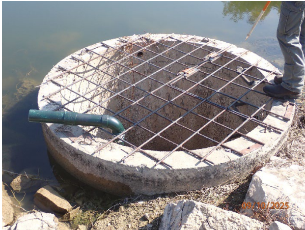
Principal spillway inlet
