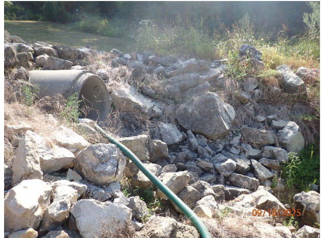
Principal spillway outlet and channel
