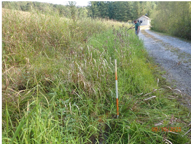
Toe – looking left (note vegetation and seepage)
