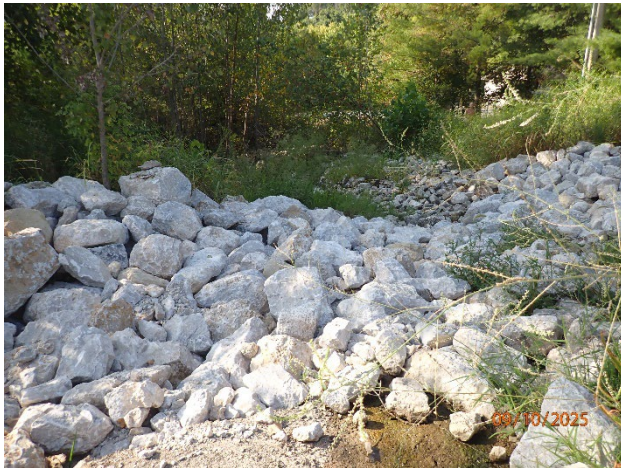
Principal spillway channel – looking downstream
