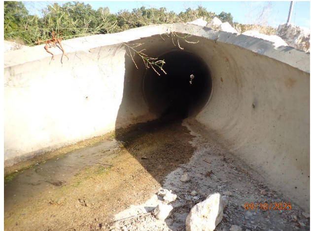
Principal spillway outlet
