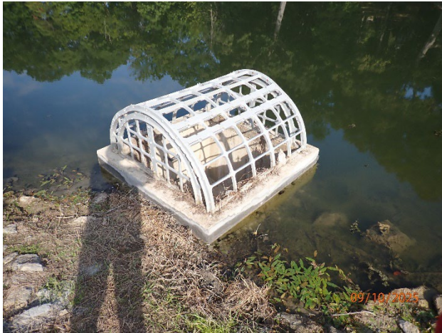
Principal spillway inlet
