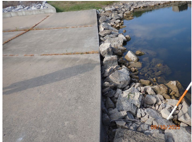
Auxiliary spillway – looking right
