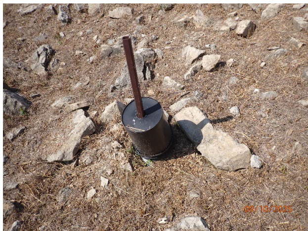
Drawdown valve pit on the downstream face
