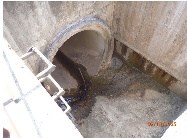
Principal spillway inlet
