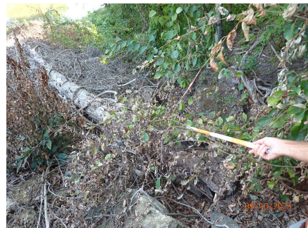
Erosion and downed tree in the right groin
