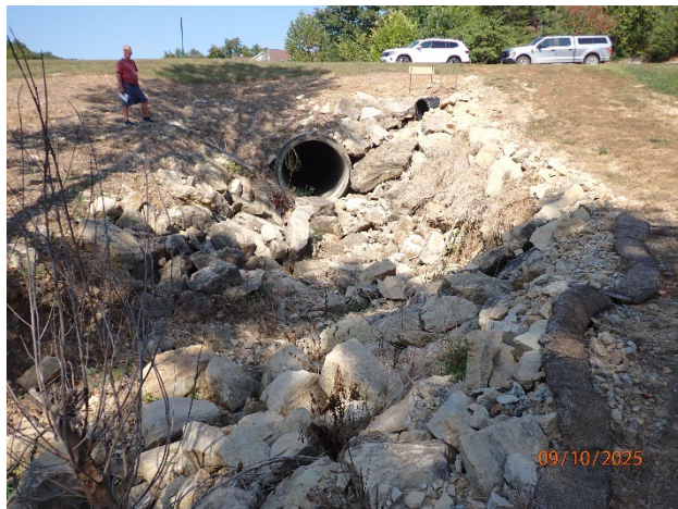
Principal spillway outlet pipe and channel – looking upstream
