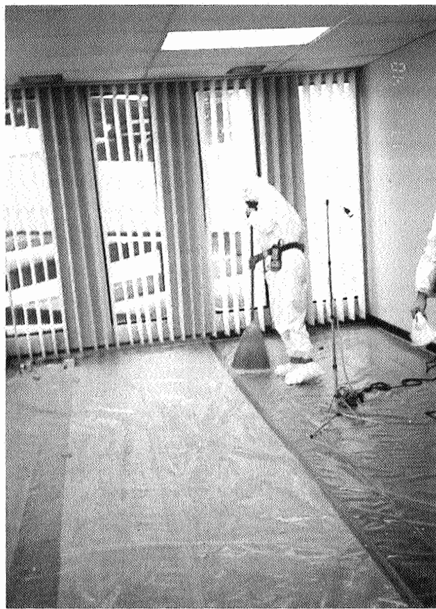
Figure 5—View of clean-up procedures with area air sampling pump at right.
