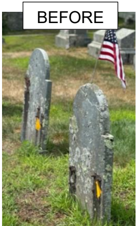
Back side of the Briggs stones showing the old iron strapping.
