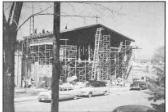
Construction work on the new St. Aloysius Church.
