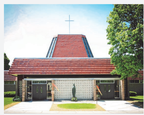
106TH STREET SITE 2322 S. 106th Street
