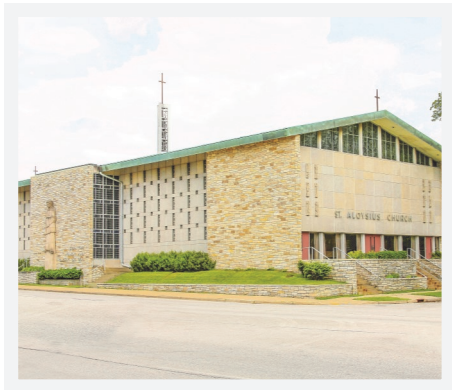
92ND STREET SITE 1414 S. 92nd Street
