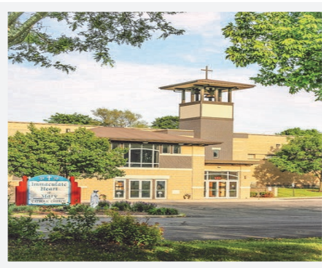
116TH STREET SITE 1212 S. 117th Street
