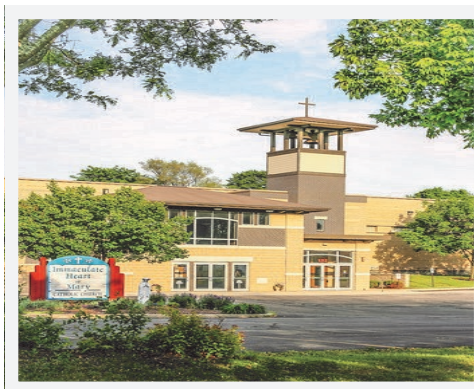
116TH STREET SITE 1212 S. 117th Street
