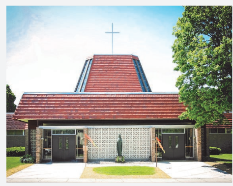
106TH STREET SITE 2322 S. 106th Street
