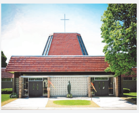
106TH STREET SITE 2322 S. 106th Street
