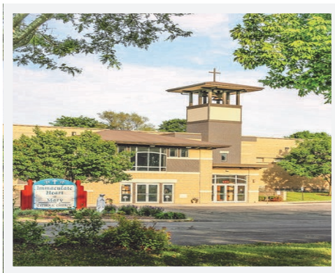
116TH STREET SITE 1212 S. 117th Street
