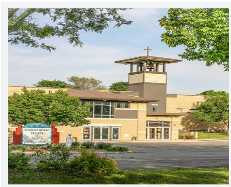
116TH STREET SITE 1212 S. 117th Street
