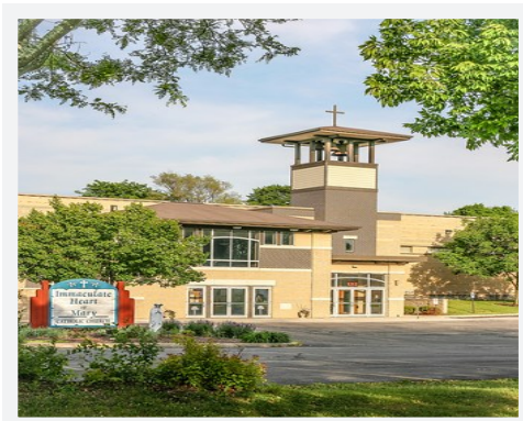
116TH STREET SITE 1212 S. 117th Street
