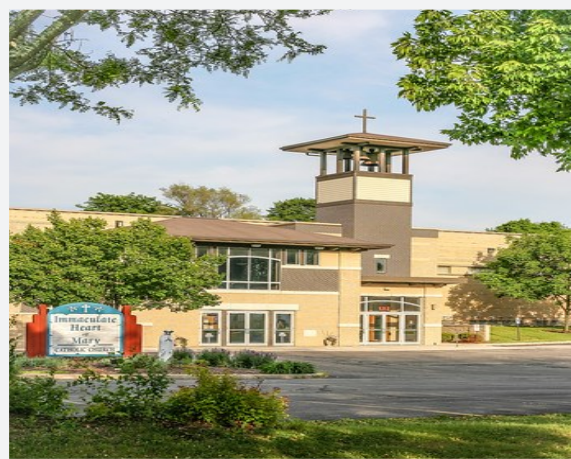
116TH STREET SITE 1212 S. 117th Street
