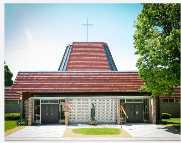
106TH STREET SITE 2322 S. 106th Street
