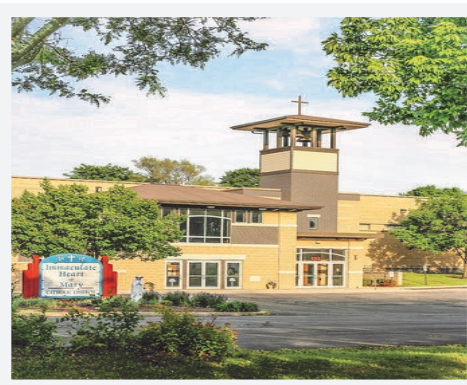
116TH STREET SITE 1212 S. 117th Street
