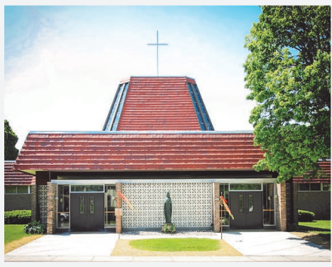
106TH STREET SITE 2322 S. 106th Street
