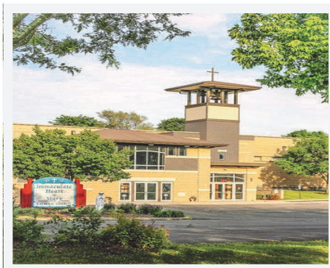
116TH STREET SITE 1212 S. 117th Street
