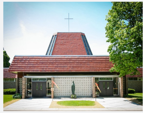
106TH STREET SITE 2322 S. 106th Street
