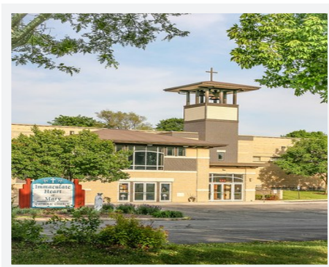
116TH STREET SITE 1212 S. 117th Street
