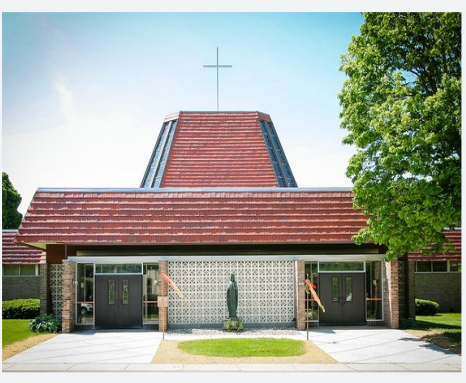
106TH STREET SITE 2322 S. 106th Street
