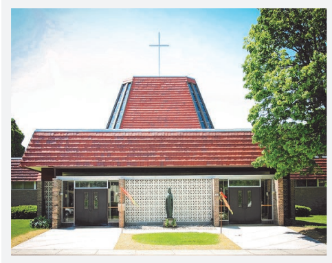
106TH STREET SITE 2322 S. 106th Street
