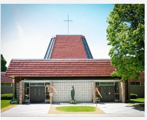
106TH STREET SITE 2322 S. 106th Street
