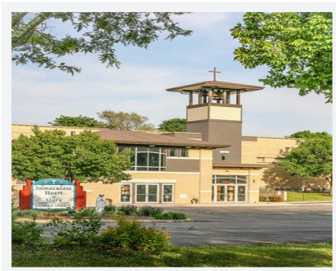
116TH STREET SITE 1212 S. 117th Street
