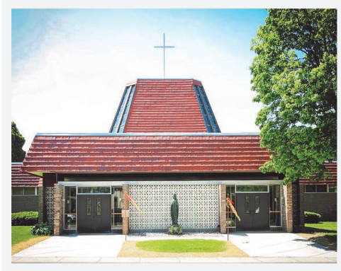
106TH STREET SITE 2322 S. 106th Street
