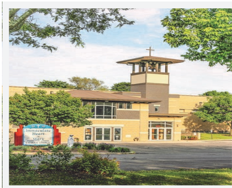
116TH STREET SITE 1212 S. 117th Street
