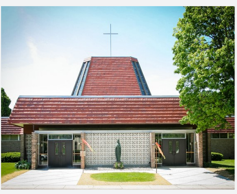
106TH STREET SITE 2322 S. 106th Street
