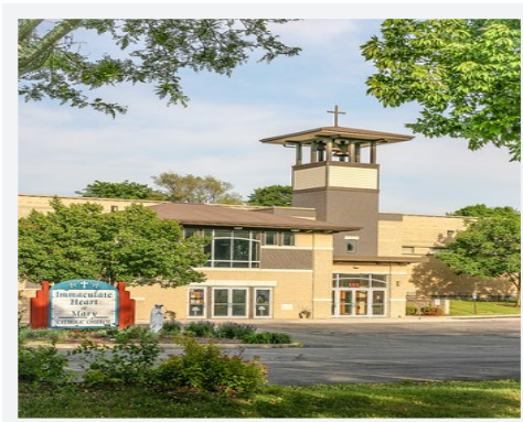
116TH STREET SITE 1212 S. 117th Street
