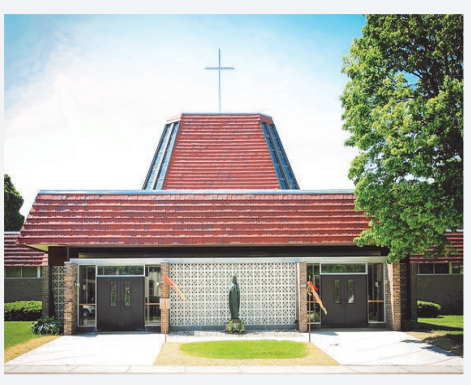
106TH STREET SITE 2322 S. 106th Street
