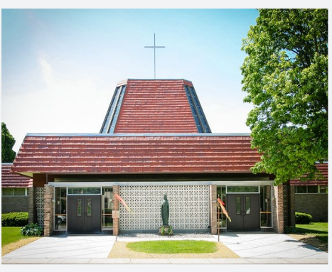
106TH STREET SITE 2322 S. 106th Street
